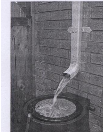
Figure. 4 : Rainwater collection (through downpipes and sieves)
